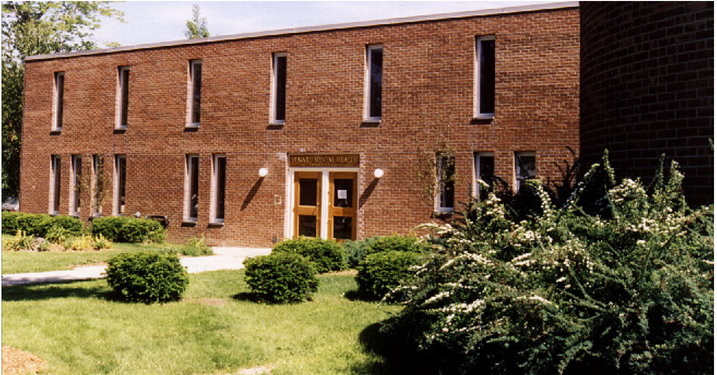
Administration Offices of Howard Community Services Flynn Avenue, Burlington, VT
