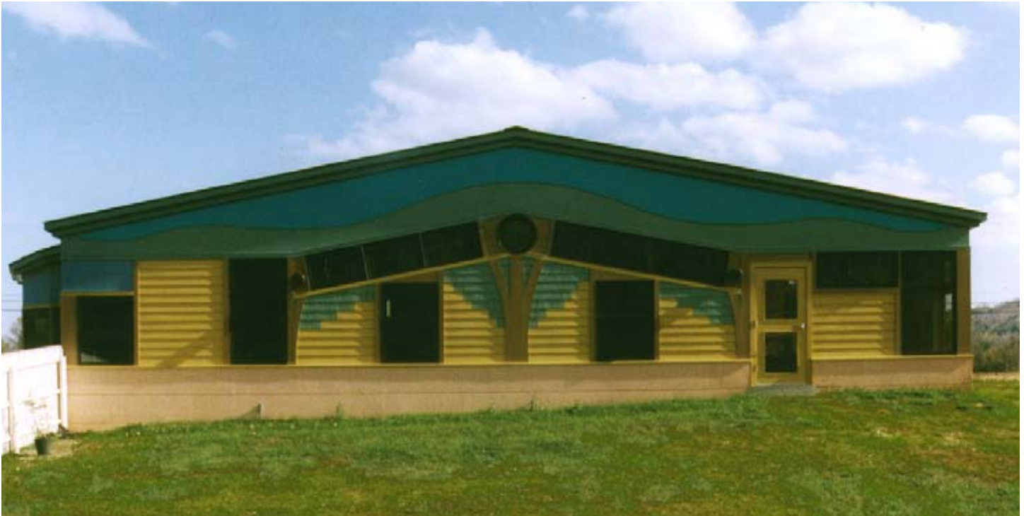
West elevation of the Bellwether School and Family Resource Center, Williston, VT
