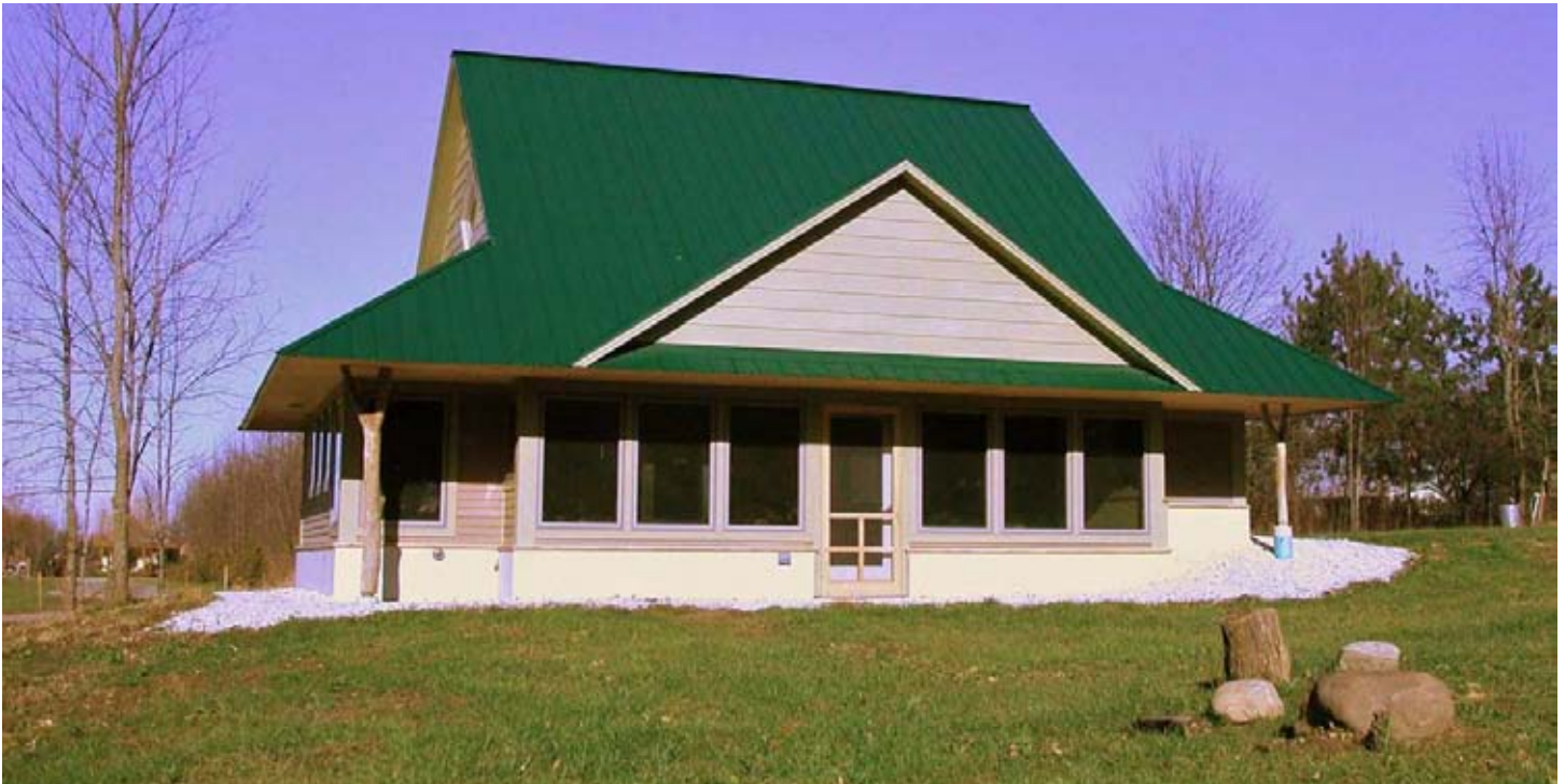
View from the southwest
